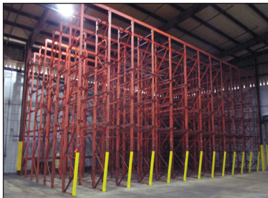
Drive-In Pallet Racking
